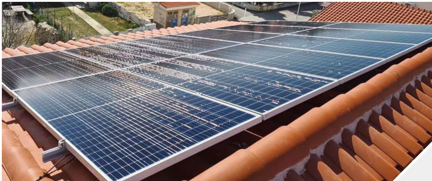
Project Address: Island Vir, Croatia Project Capacity: 8kW Inverter: 1 set of Sunways STT 10kW inverter
